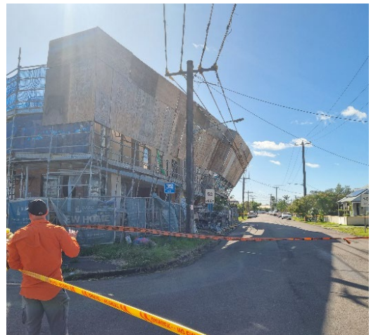
Scaffolding looking east
