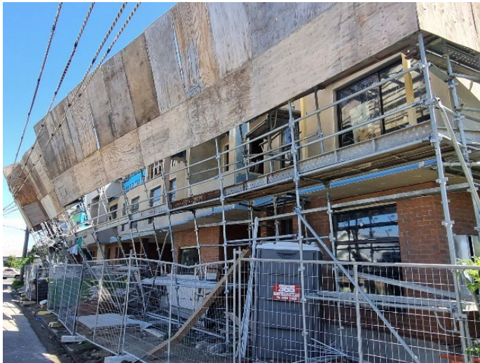
Scaffolding looking west
