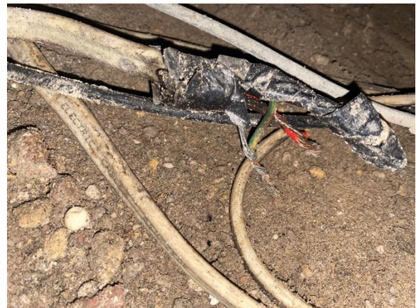
Incident site underneath the house where exposed electrical cables were located.
