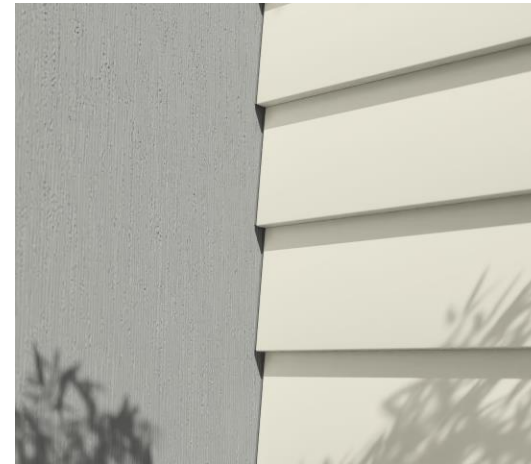
PANEL TO WEATHERBOARD - INTERNAL CORNER VERTICAL JUNCTION CAVITY FIX
